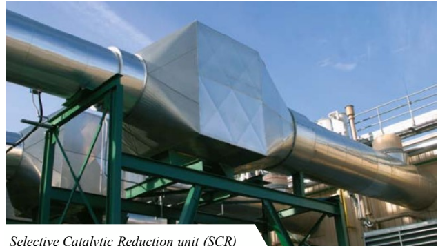
Selective Catalytic Reduction unit (SCR)
